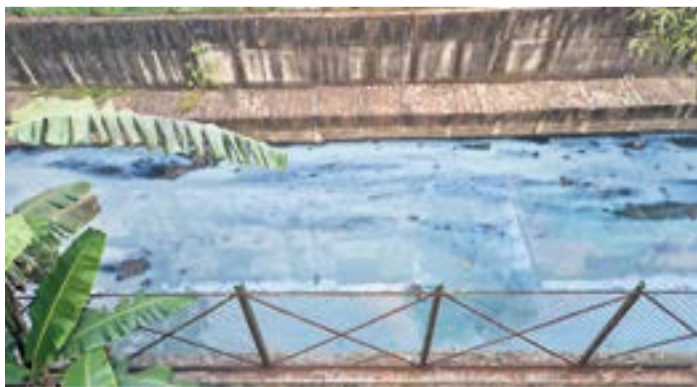
Untreated waste is systematically dumped into the canal after 8 a.m.
