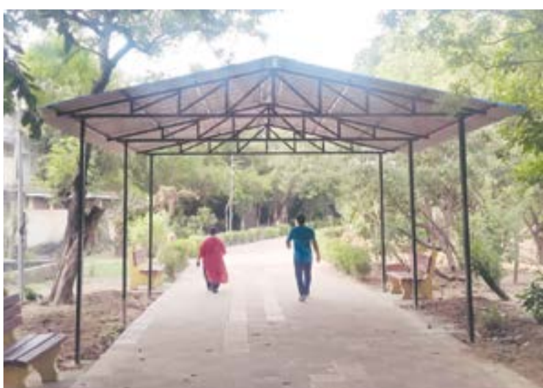
A high raised shed is put up on the east and west sides of the walking track at Mangal Eri Park in Mogappair. This has been erected to shelter the daily walkers from a sudden downpour during rainy season.
